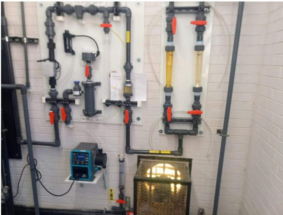
Pictured is the generator that UBT's Water Treatment Plant is using to conduct a trial study using chlorine dioxide as a pre-oxidant. To date, compliance test results for TTHM's and HAA5's (disinfection by-products- aka DBP's) have been significantly reduced as evidenced by fourth quarter 2019 test results.
